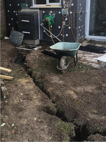
Above is a picture of the connecting trench to the manhole, done mainly by hand, as the main sewer is situated around this area. Over the years many buried things have been "discovered", and I had no wish to "discover" the sewer pipe with the trencher! Prior to trenching, "linesearch before u dig" were contacted, who will give a free check for homeowners to see what is there. Our back garden is happily free of any high voltages or phone lines or water or gas.
