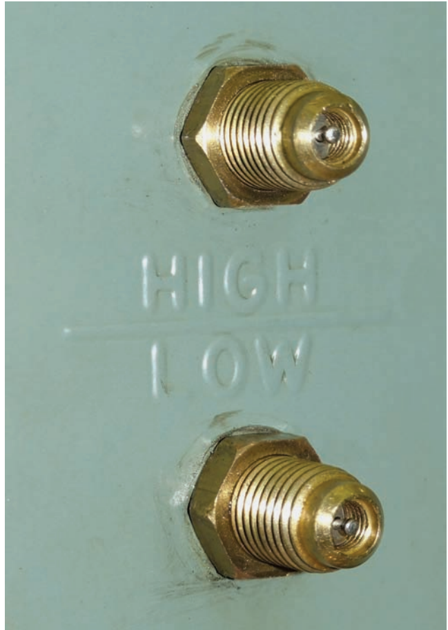
Figure 25-7 High side and low side Schrader valves on a packaged unit
