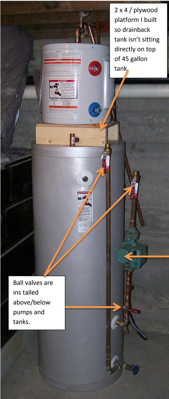
2 x 4 / plywood platform I built so drainback tank isn't sitting directly on top of 45 gallon tank.
