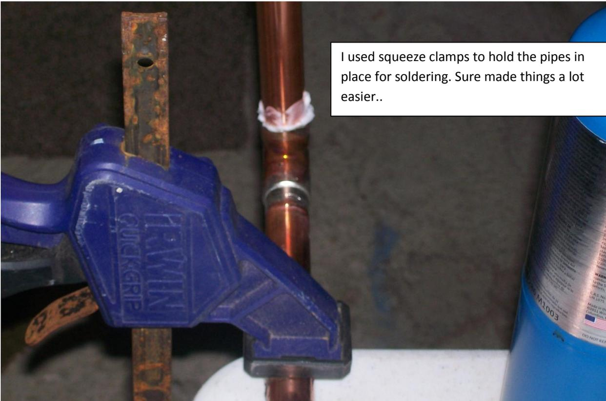
I used squeeze clamps to hold the pipes in place for soldering. Sure made things a lot easier..
