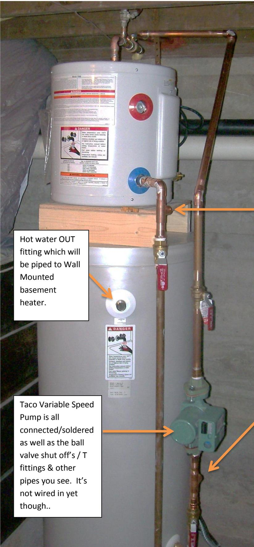
Ok.. Most everything is in place and connected now except for installing the sight glass on the drainback tank. I installed another storage tank with built in heat exchanger for domestic hot water use to the RIGHT of the 2 tanks you see in the picture.
