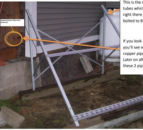
This is the rack that holds the evacuated tubes which will be mounted on the roof or right there where you see it on the ground bolted to 8 x 8 pressure treated.
