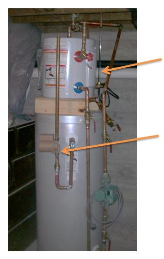
This is a picture of the drainback tank and 45 gallon Superstor storage tank used for heat distribution.
