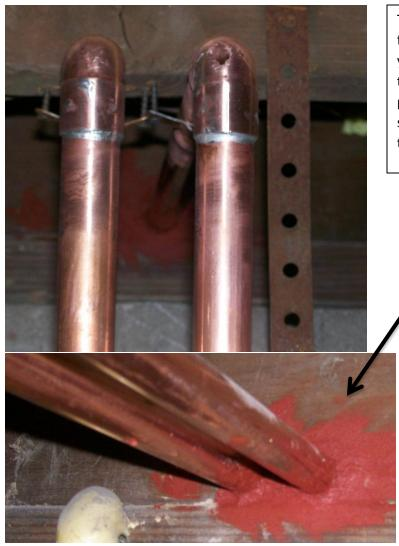
This is the supply/return ¾ pipes attached to floor joists. If you look behind the elbows you'll see where they go out thru the side of the house. The hole openings around the pipe are sealed with high heat furnace type silicone. Take a look at next picture to see the silicone..
